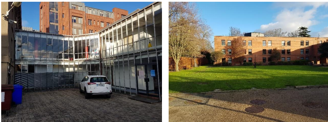
Figure 2 - View of Existing Sports Hall and Cunningham House at Trinity Hall
